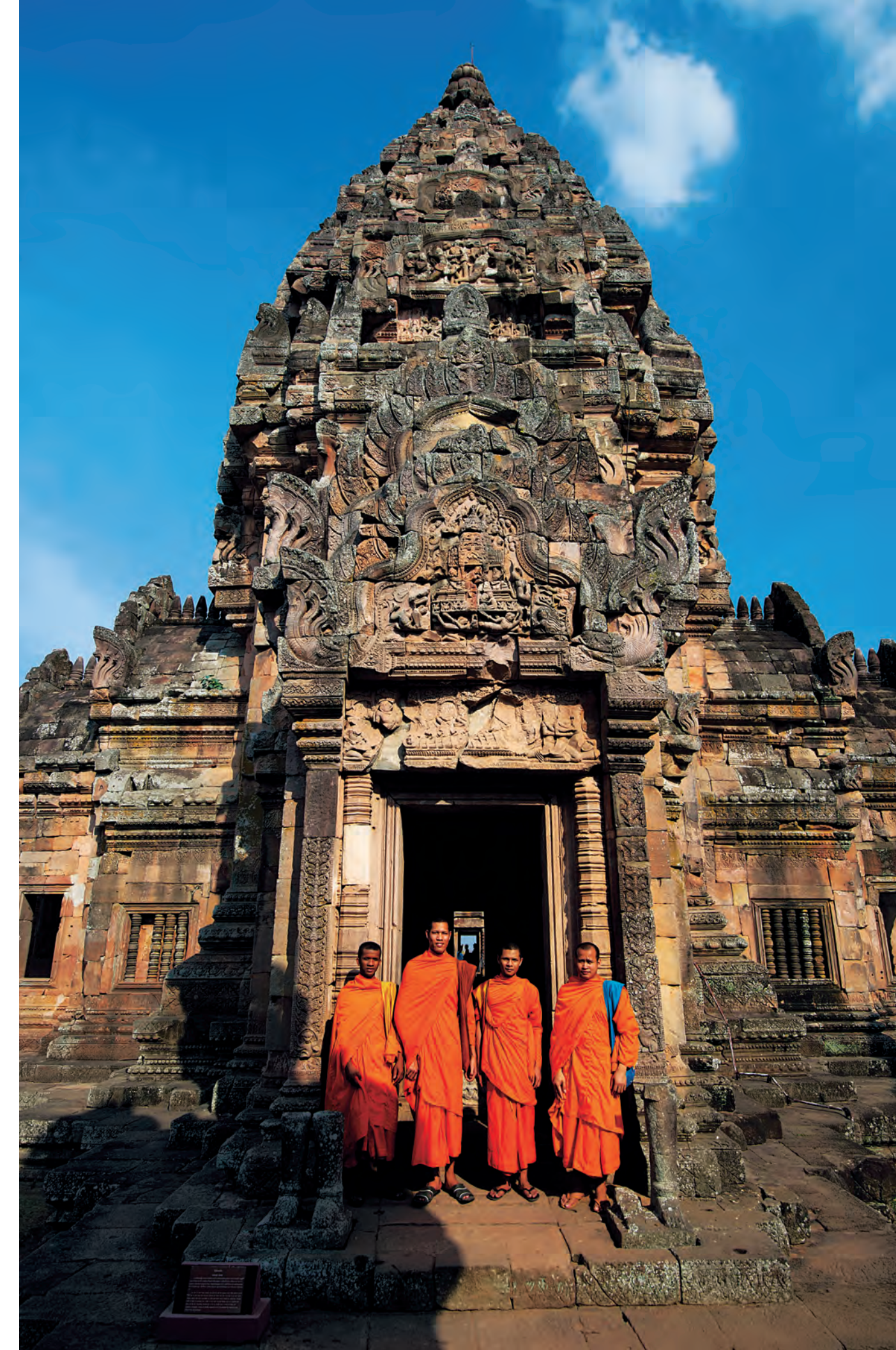
On top of an extinct volcano of Buri Ram is the location of Prasat Phanom Rung, a pink sandstone castle, attractively decorated and constructed as a dedication to Shiva, the supreme god of Brahmanism. The Prasat reflects the greatness of the ancient Khmer civilisation through various details of the structure and decorations.
