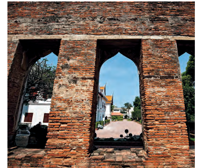
Top Chanthara Phisan Hall of Thai architecture was used as an audience hall of King Narai the Great and as an administration centre. After it was abandoned, the Hall was in a state of ruin until King Mongkut (Rama IV) restored it to be the condition as can be seen at present.
