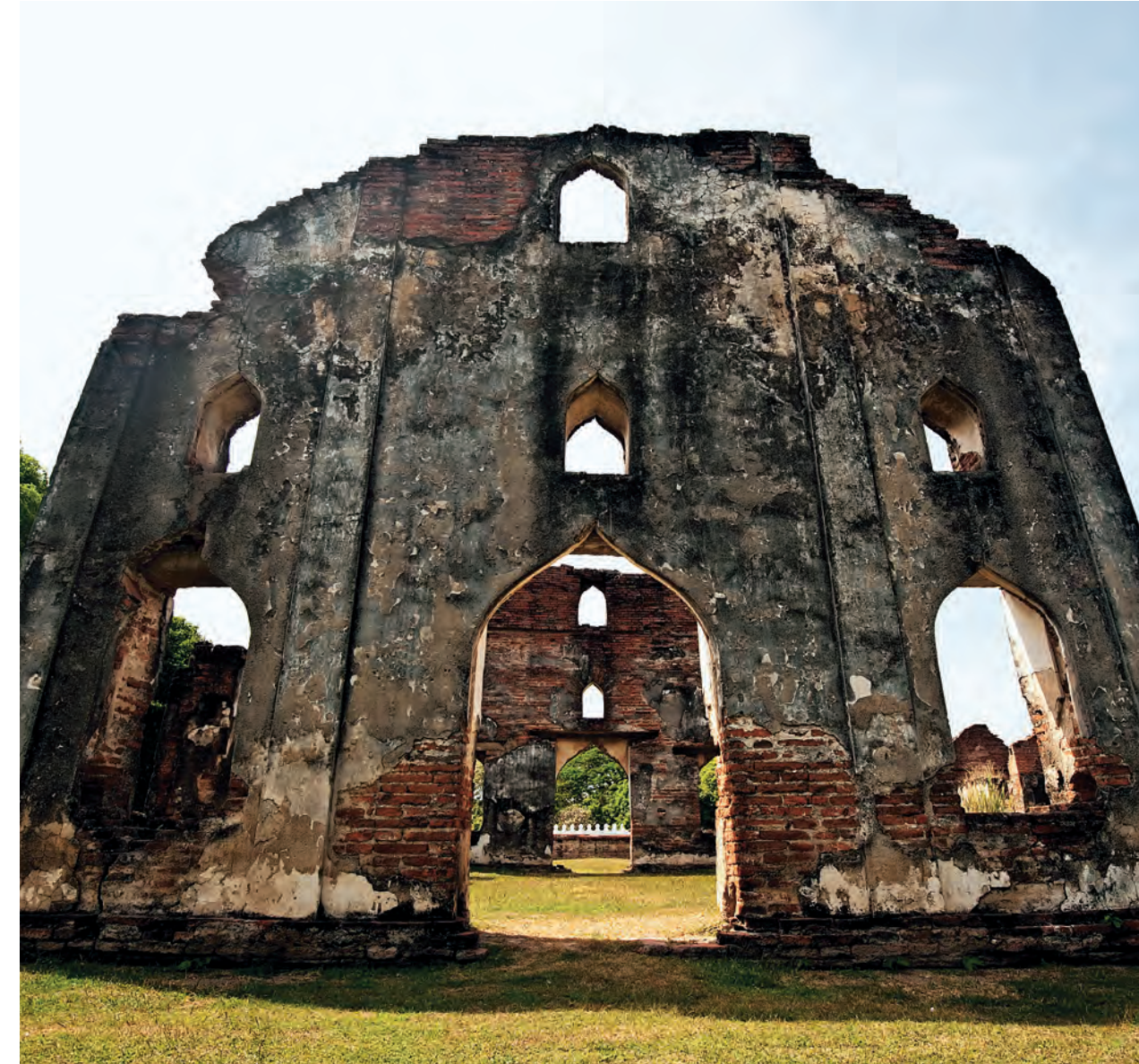
Left and Right The condition of the structure of the building that welcomed international diplomatic corps after many hundreds of years had passed.
