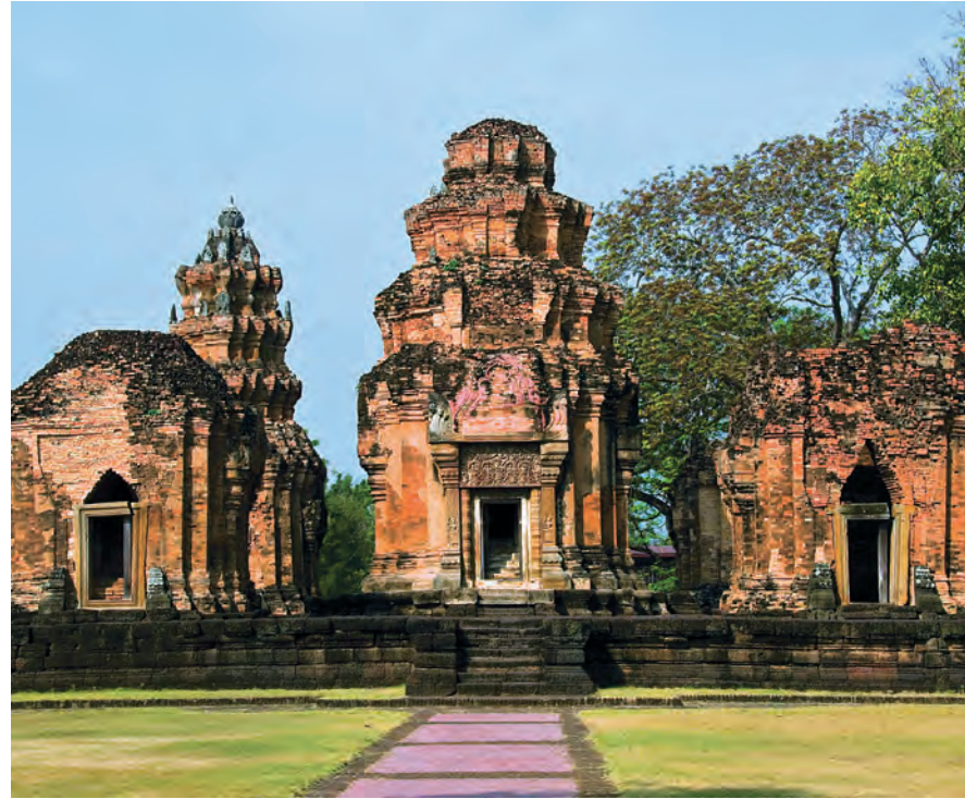
Prasat Sikhoraphum is a prasat with 5 chedis of brick without mortar on a laterite base. It has a moat on 3 sides and is the best planned ancient stone prasat to study.
