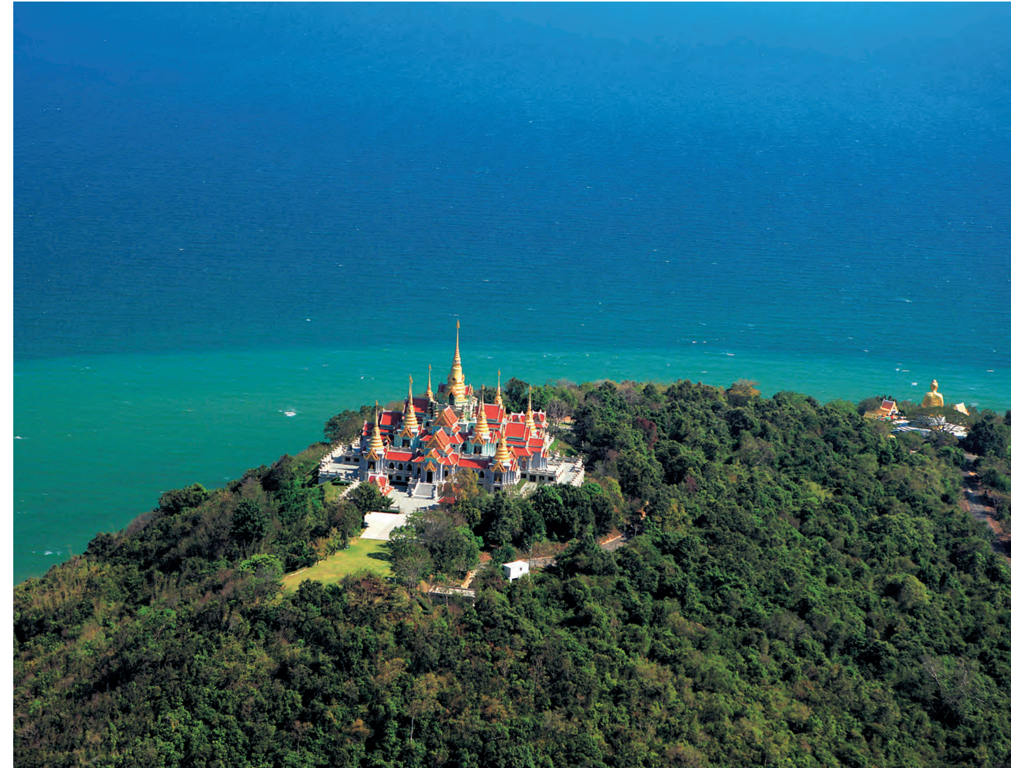
The Chalemongkolasana Residence and Mareeraja Rattabanlang Residence are located in the grounds of Sanam Chandra Palace, Nakhon Pathom. They were constructed during the reign of King Vajiravudh (Rama VI) with the inspiration from Chenonceau that is located on the bank of the Cher River, France. They comprise two buildings built to cross the river in which there is a bridge linking the two buildings. They are made in the early Renaissance architectural style and adapted to the climatic conditions of Thailand.
