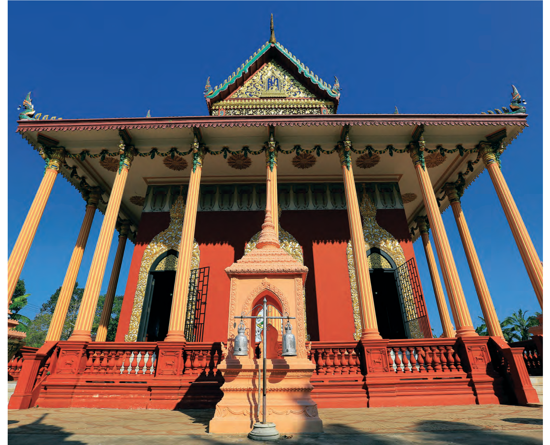
The ubosoth of Wat Kaeo Phichit, Prachin Buri province was constructed in the reign of King Rama V the Great. It is a distinctive building that is the only one of its kind in Thailand, as it has a combination of 4 architectural styles: Thai, Chinese, Western, and Khmer. The plan of the ubosoth, door panels, windows, gable apex, the tooth like ridges on the sloping edges of the gables, and swan’s tails are Thai; the staircase rail, the triangular dragon designs, and roof are Chinese; the Corinthian pillars and the paintings of Westerners around the ubosoth are Western, and the defensive wall and arches are Khmer.
