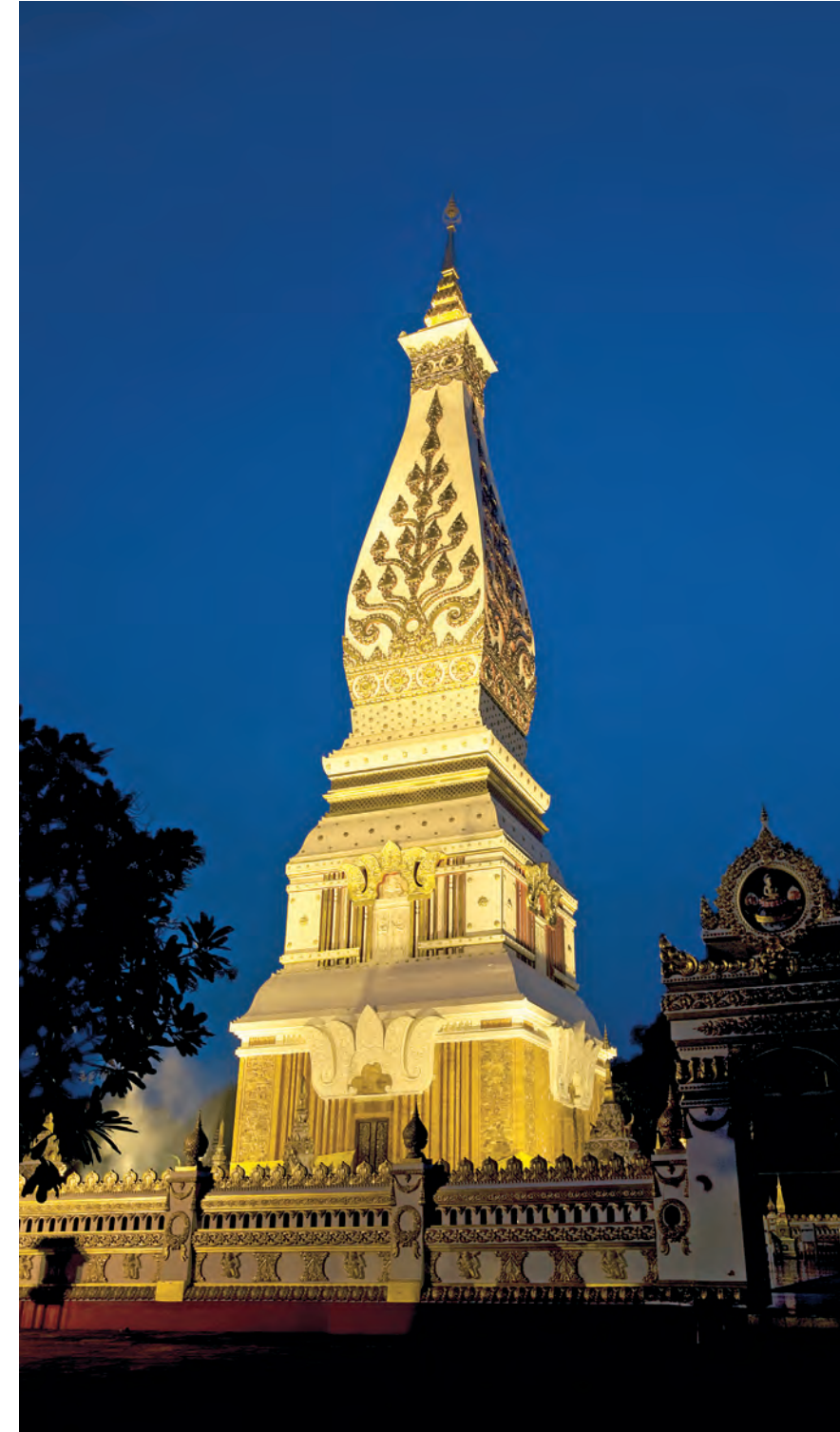
The antiquity and sacredness of Phrathat Phanom is the thing that reaffirms the faith of the Buddhists along the bank of the Mekong River. The Phrathat was constructed by brick on a square base with the top having carved designs of a Si Maha Phot tree as well as covered with gold and decorated with beautiful gems.
