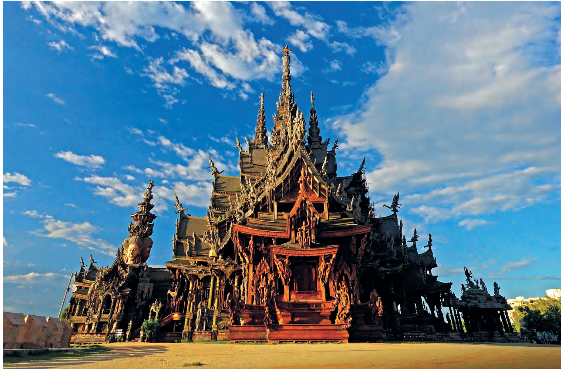
The Sanctuary of Truth, Chon Buri province is a structure entirely made of carved wood and the largest one of its kind in the world. The top of the Sanctuary has four open porticos, the roof overlaps on all four sides, and the entire structure is decorated with carved wooden sculptures combined with stunning Thai decorations and architecture from the Early Ayutthaya Era to the Rattanakosin Era.
