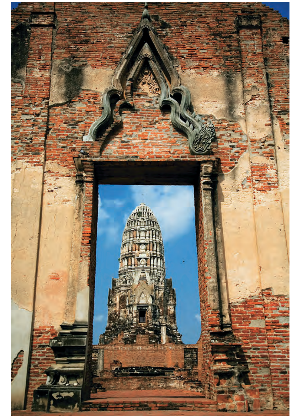
Wat Ratchaburana is an ancient temple built during the Early Ayutthaya Era of the reign of King Samphraya. In the centre of the temple is a Thai style prang that is admired for its high base. The front of the prang has a large portico extending out like a booth. The top tapers into a high tip like a corn pod that has a nine-tiered stupa. Under the prang of this temple is where you could see numerous beautiful royal objects and art made of gold. At present, they have been kept in the Samphraya National Museum.
